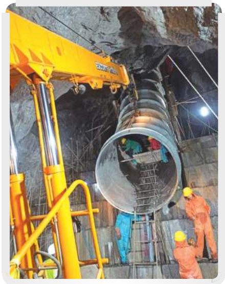
Penstock Pipe Installation
