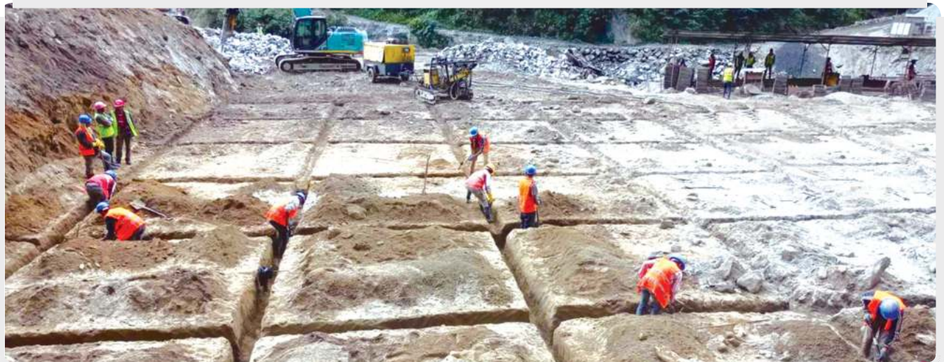
Excavation of Trench at Switchyard
