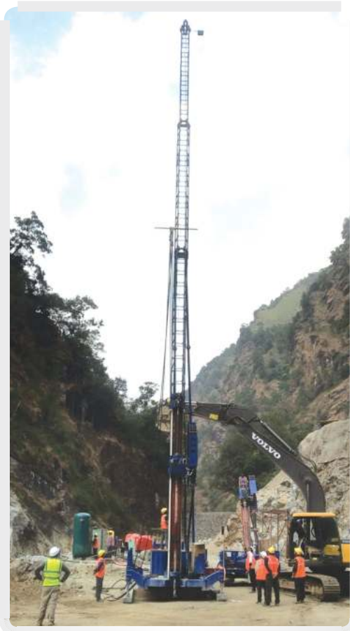
Jet Grouting at Headworks
