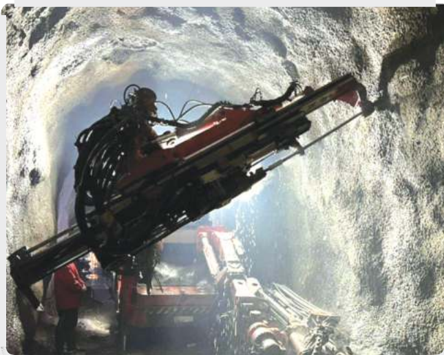
Drilling Works at Headrace Tunnel
