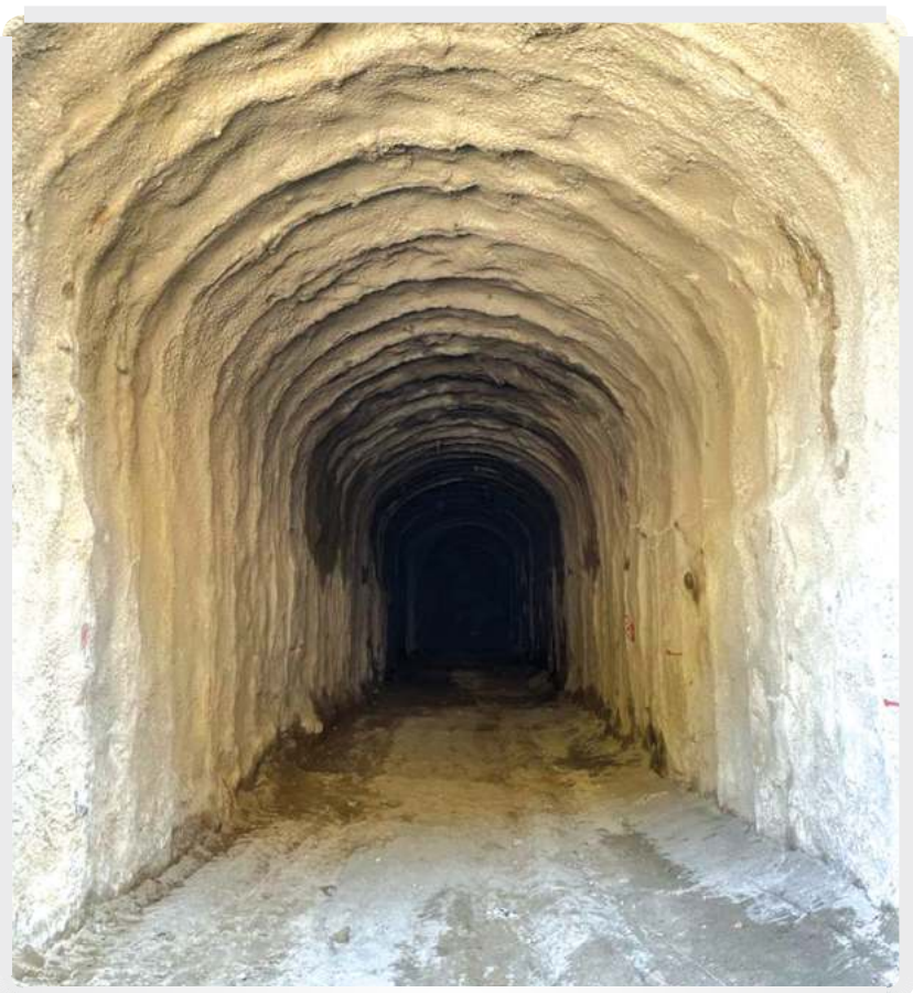
Left Bank Grouting Tunnel
