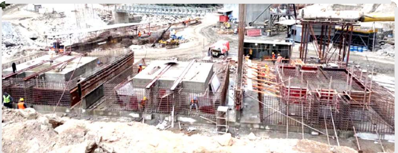
Transformer Foundation Rebars and Concrete Works
