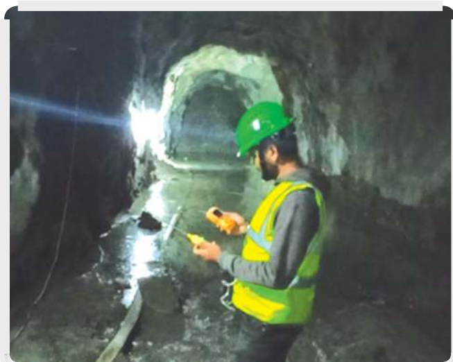
Gas Monitoring inside Tunnel
