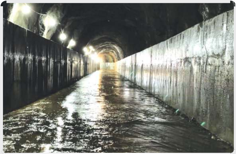
Diversion Tunnel After Lining
