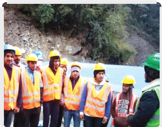
Toolbox and Safety Training at Site
