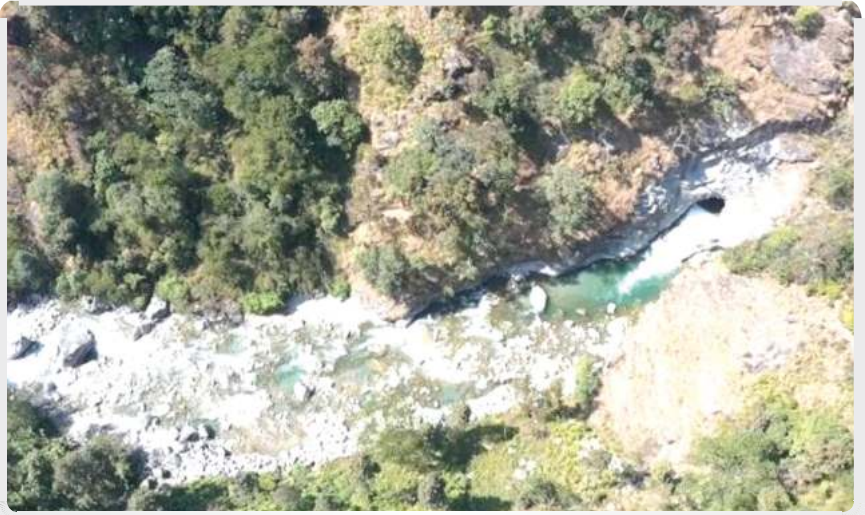
River Diversion Tunnel-Outlet
