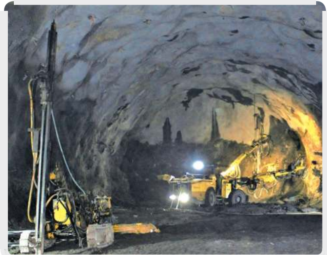
Boomer use at Powerhouse Caver
