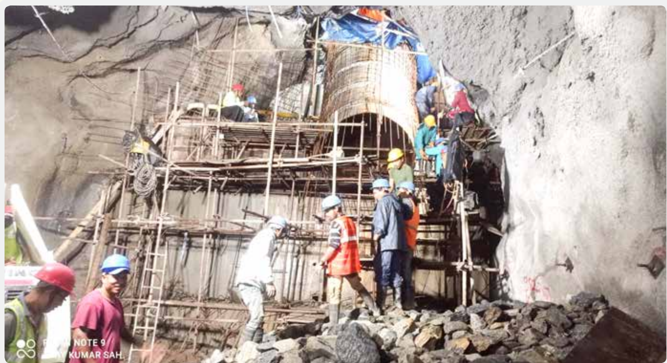
Concreting Works at Anchor Blocks
