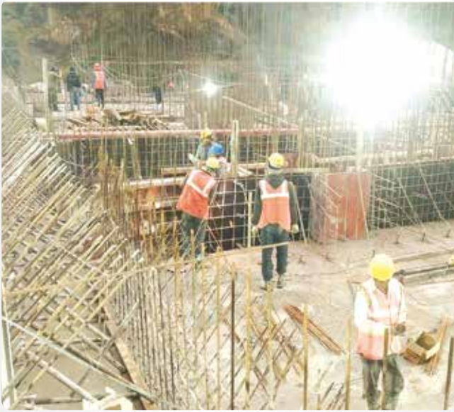
Construction of Headpond
