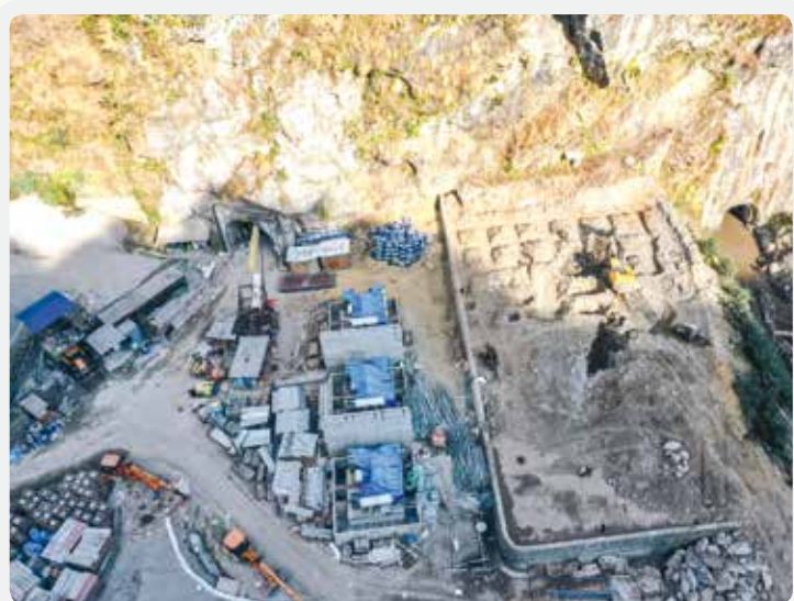
Powerhouse Area Overview
