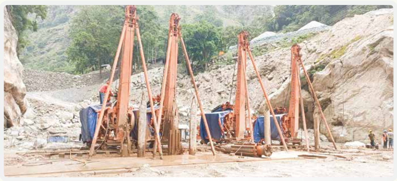
Cut-off Wall Construction
