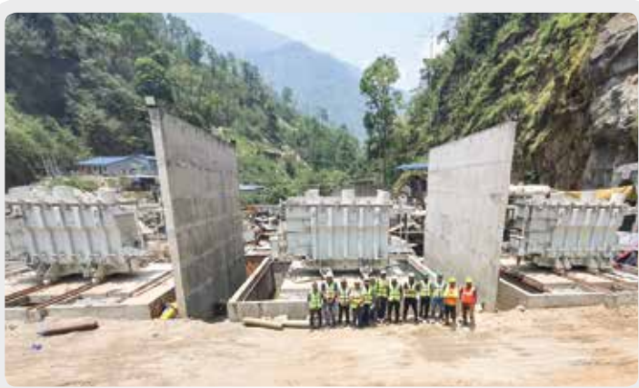
Switchyard Transformer Installation Completion
