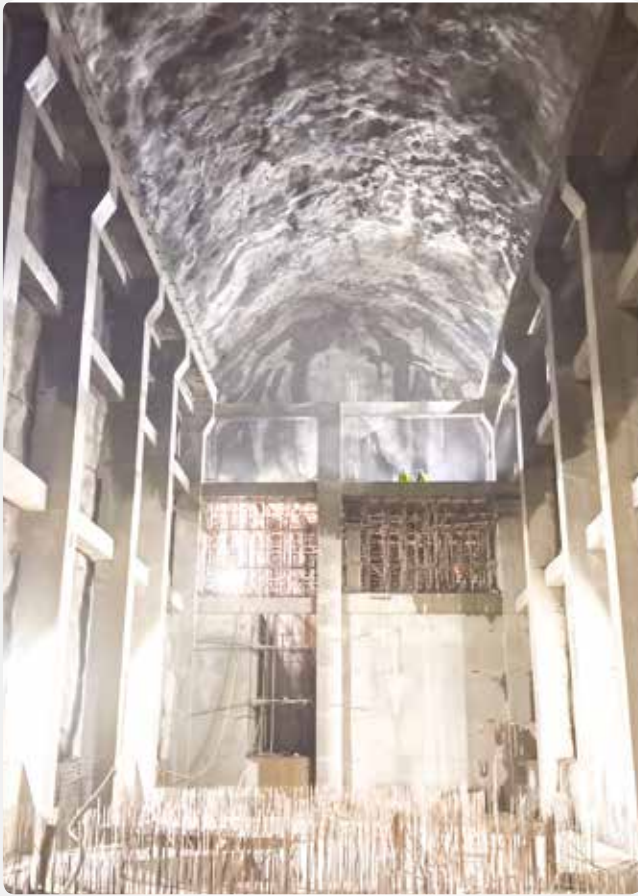
Powerhouse Control Room
