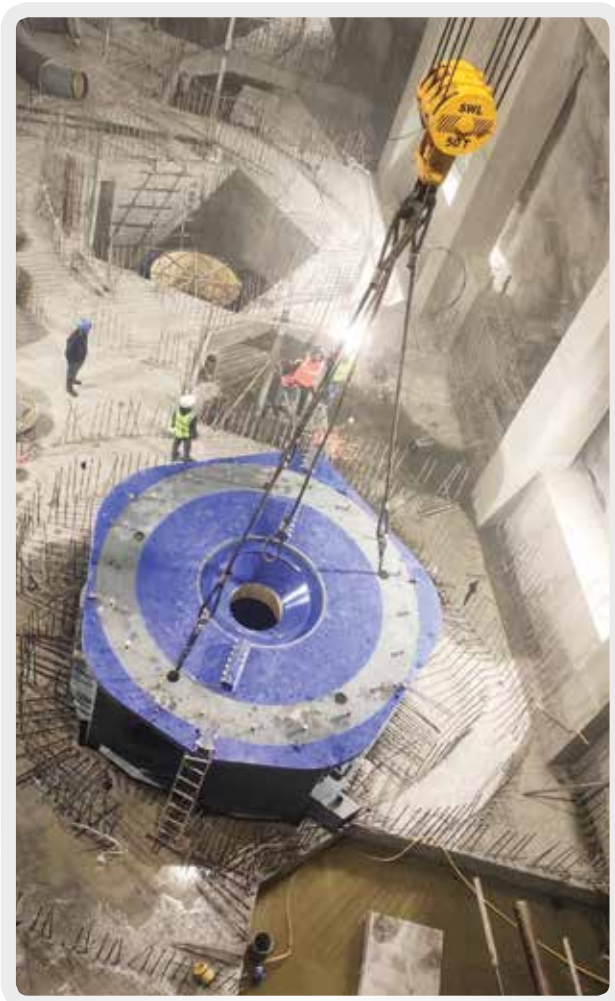
Turbine Housing Installation at Powerhouse
