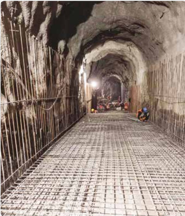
Rebar Works at Tailrace Tunnel
