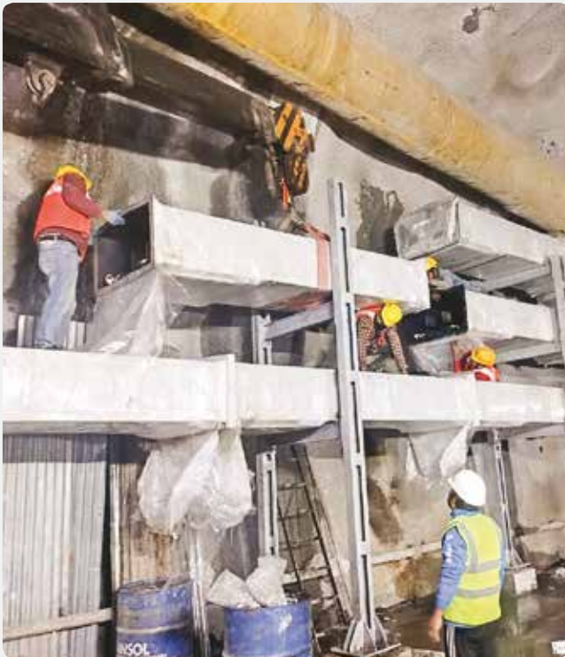
Bust Duct Installation
