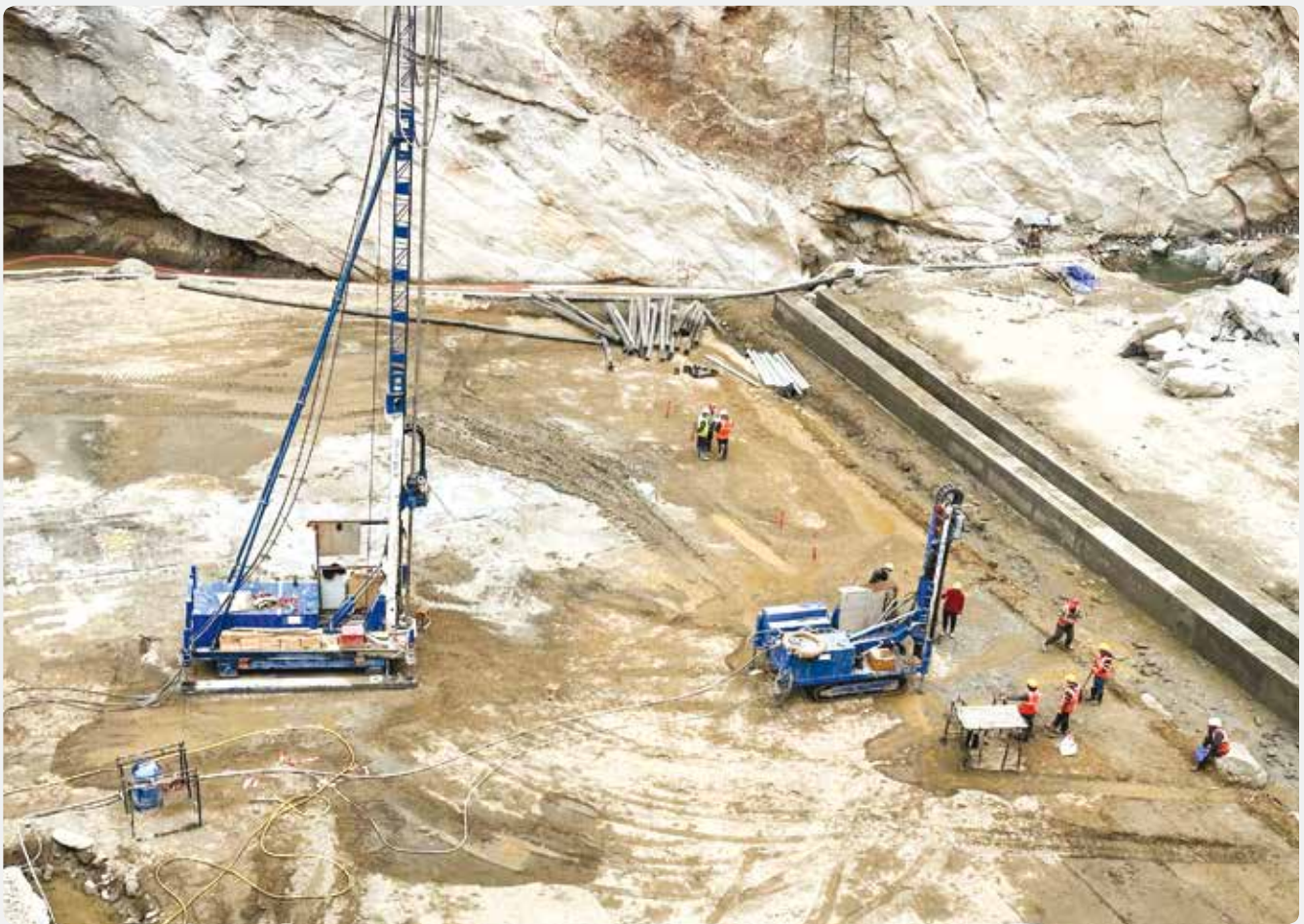
Jet Grouting at Headworks
