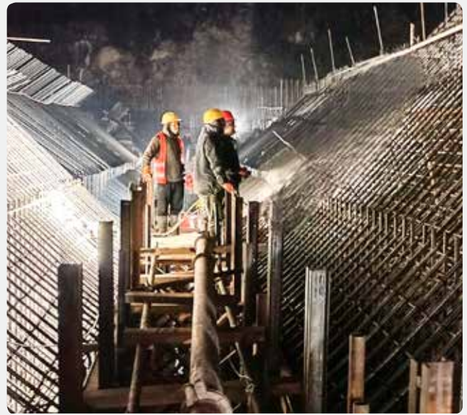
Construction of Desander
