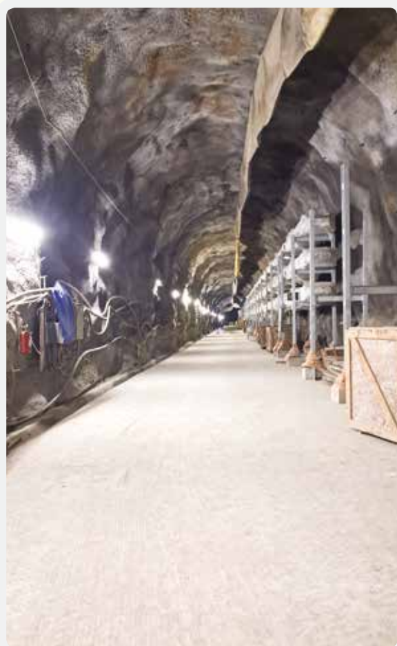
Main Access Tunnel
