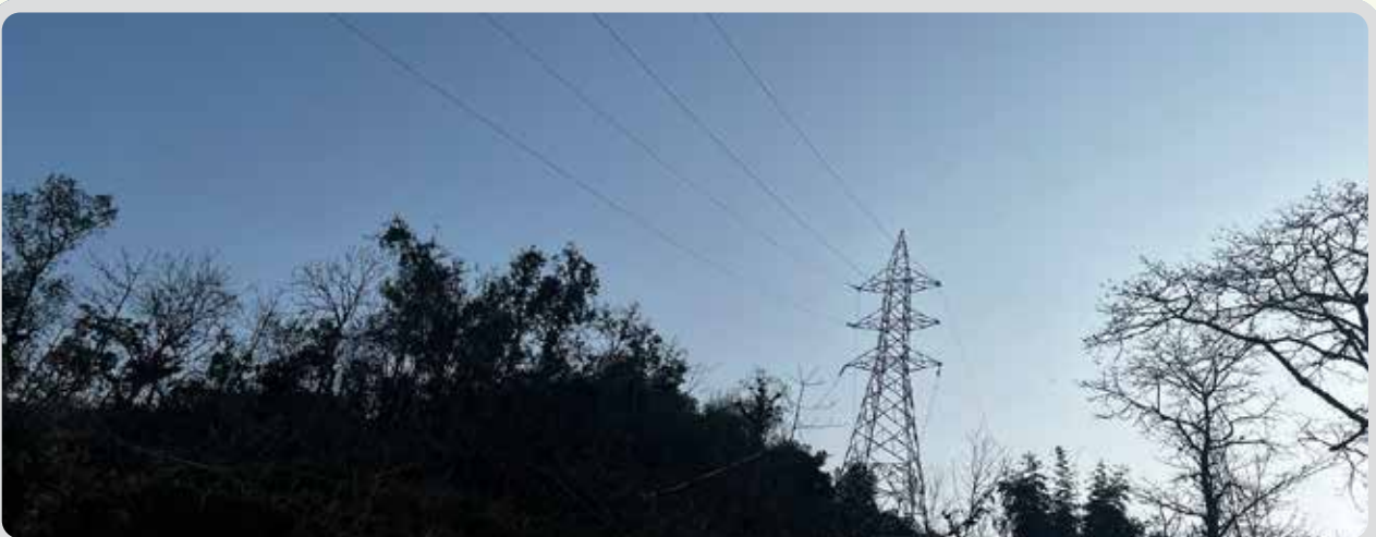
132 kV conductor stringing Ongoing
