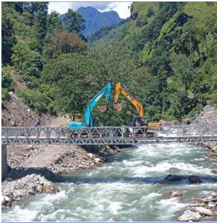
Bailey Bridge at Powerhouse
