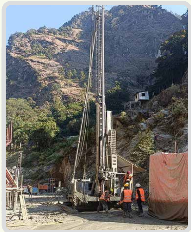
High pressure Jet grouting works
