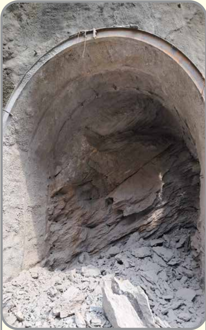
Drilling works at HRT Inlet
