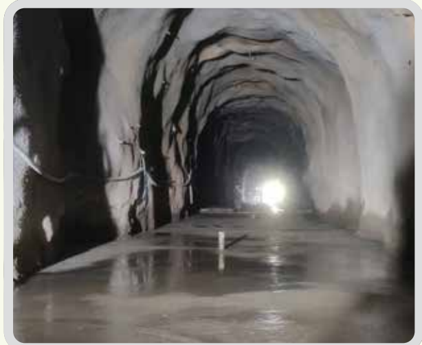
HRT Shotcrete works
