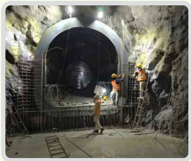
Bellmouth erection completed
