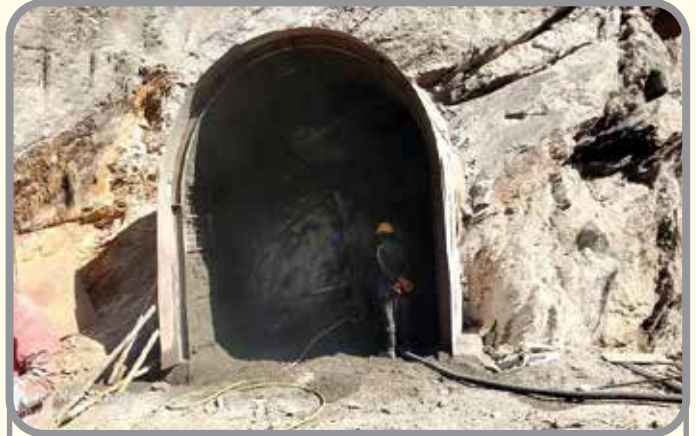
Ongoing work at Inlet Portal Canopy
