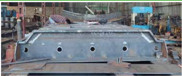
Sluice Gate Fabrication Works
