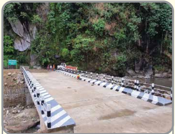
RCC Bridge Construction at Lowa Khola
