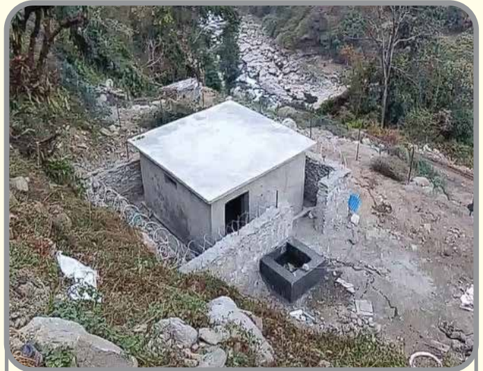
Emulsion Bunker at Headworks
