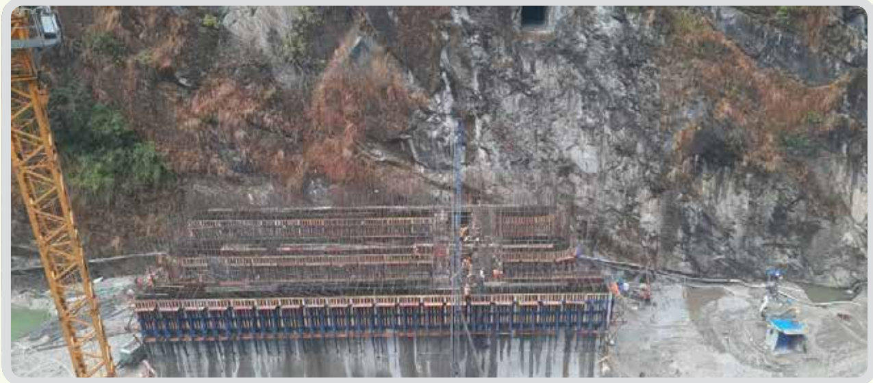
Right side Dam Ongoing concrete works
