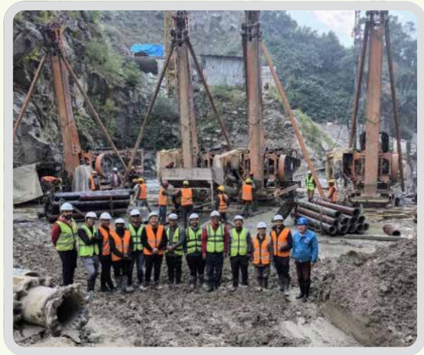
Seepage Cutoff wall at Headworks concrete work completed
