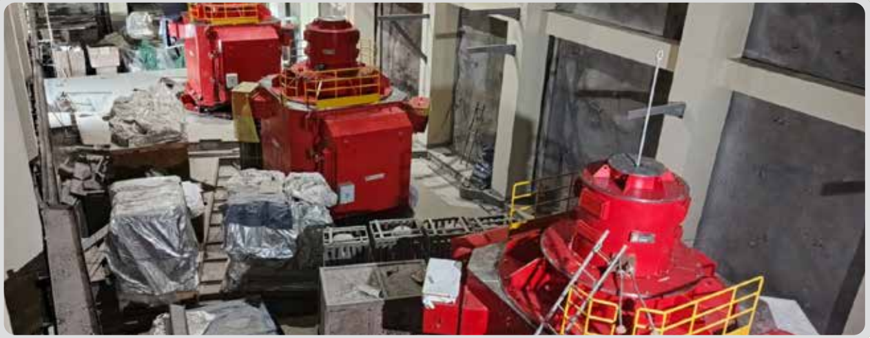
Generator Installation completed
