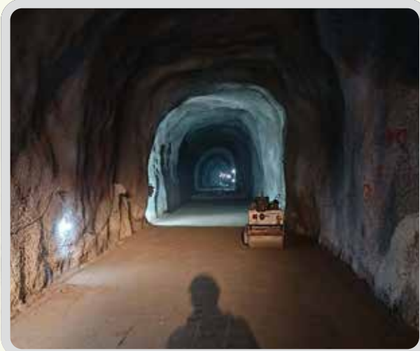
HRT Invert compaction
