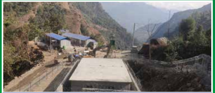
Developers Camp at Headworks Area
