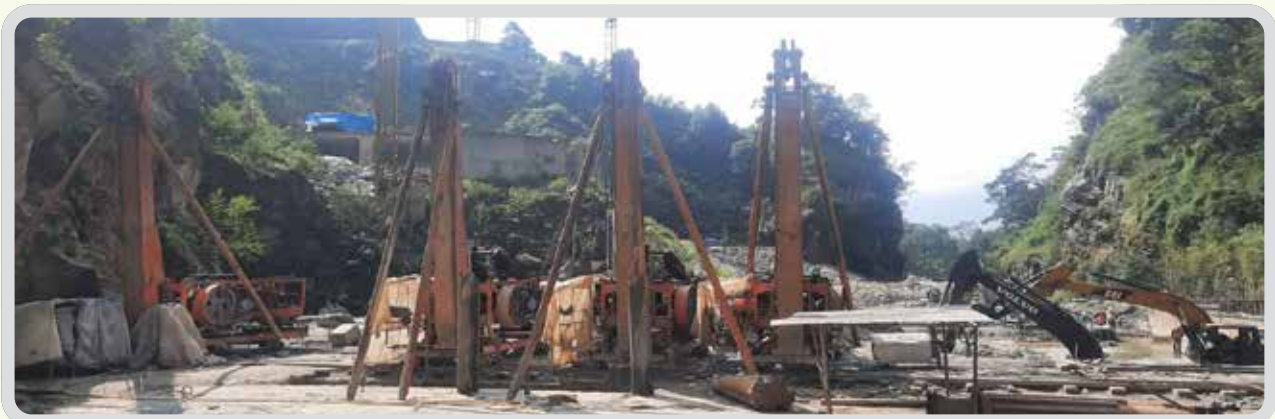
Seepage Cutoff wall at Headworks concrete work completed
